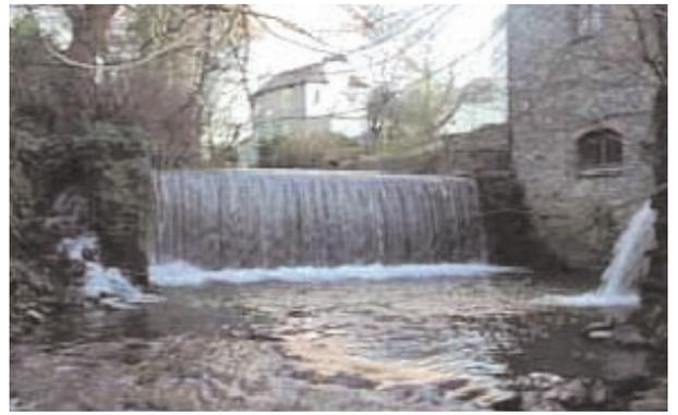
**Two complete stoppers: A weir on the Gavenny and a pipe bridge on the Ethrim. Allowing access upstream of these barriers will increase both salmon and trout production. They are priorities for action.**
