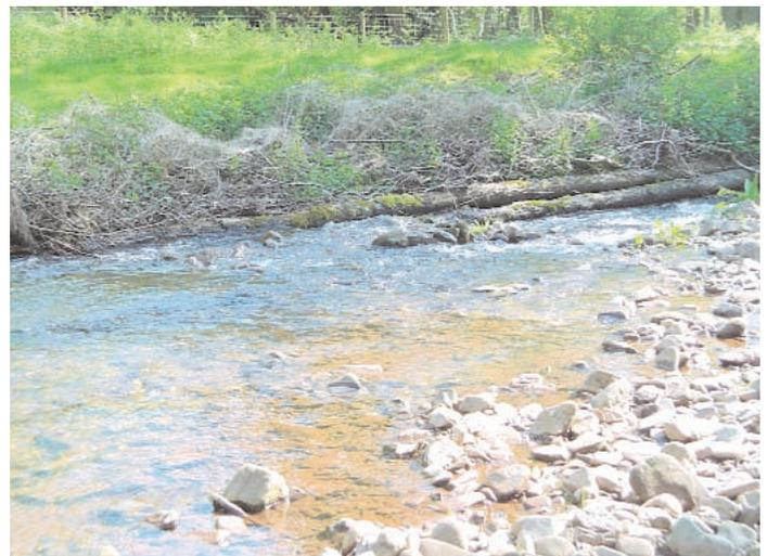
*A soft revetment on the Rhiangoll installed in 2005, that has arrested erosion and is providing good cover*
